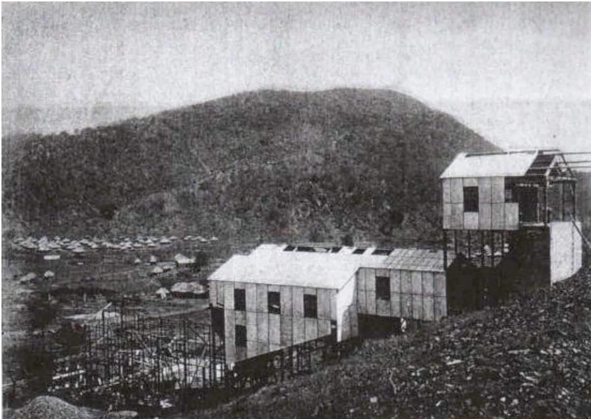
First mill erected at Penge, north of Lydenburg, during 1928/9 (Photo: Dr. Hall)
