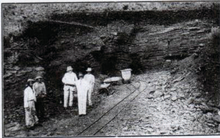
Crocidolite workings with cocopan on rails to the working face, on Oudeplaats, near Daniels Kuil
