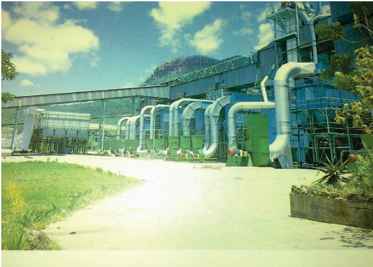
Penge mill, showing extensive modern dust-control facilities
