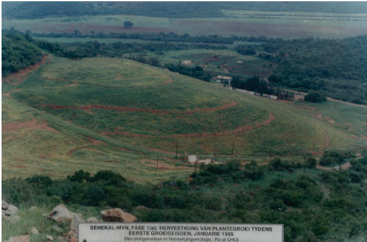
Senekal Mine dump, after reshaping and revegetation
