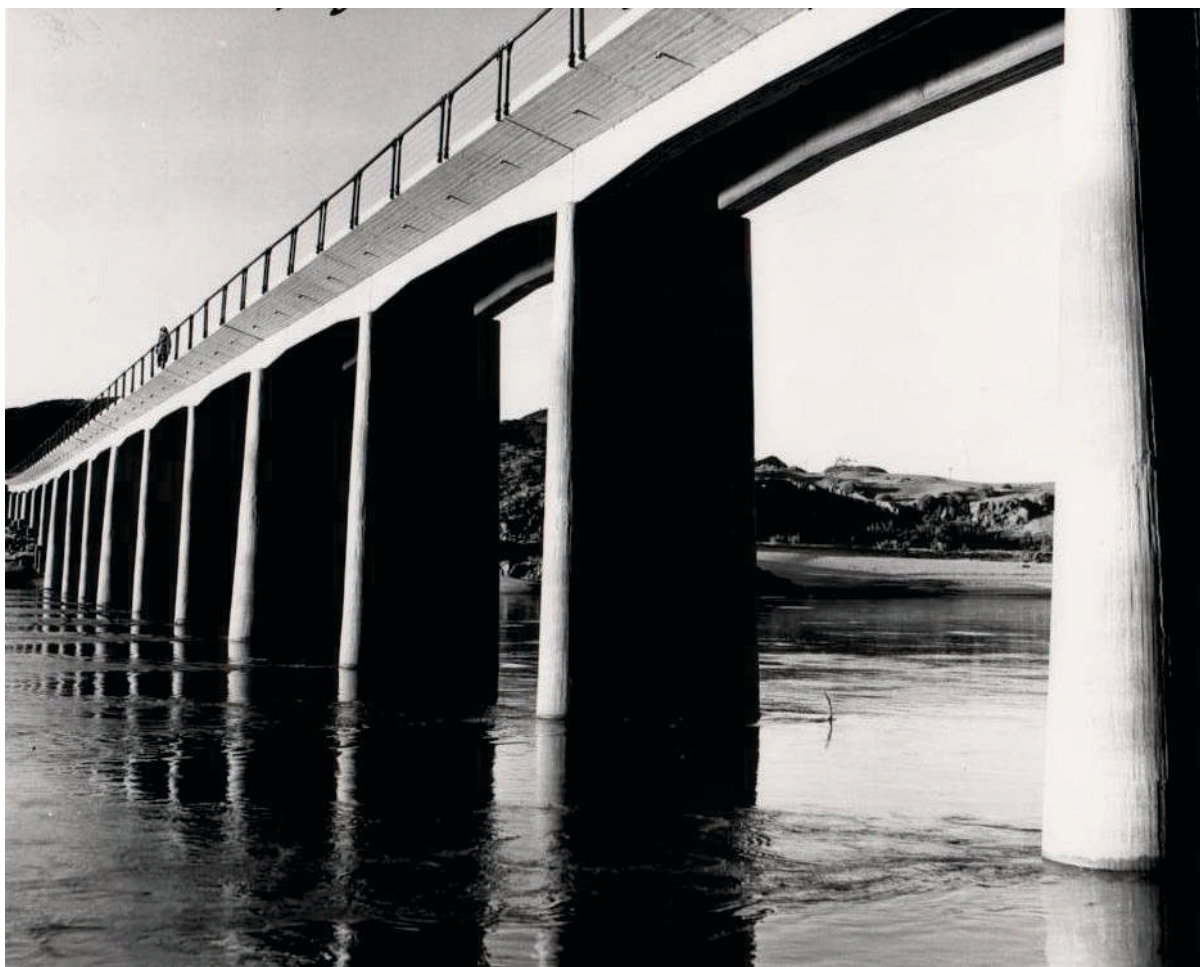
The Riley Bridge across the Orange River
