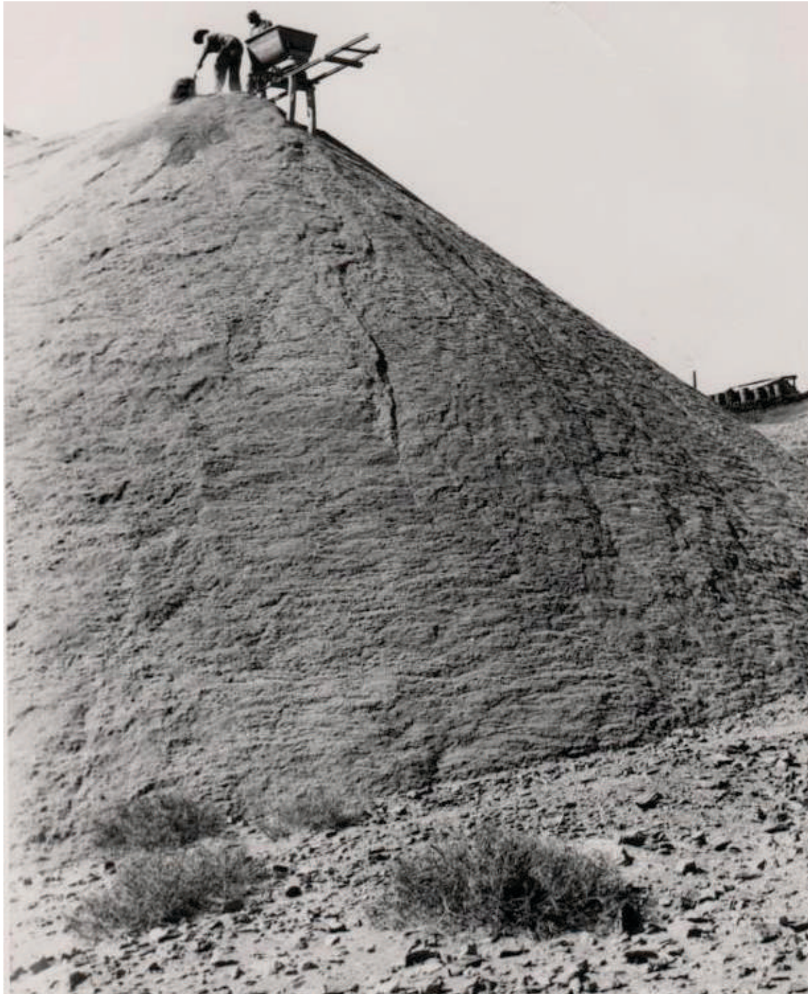
Prieska tailings dump. After the plant closed, the tailings were removed and retreated at Joyner's Stofbakkies operation across the Orange River
