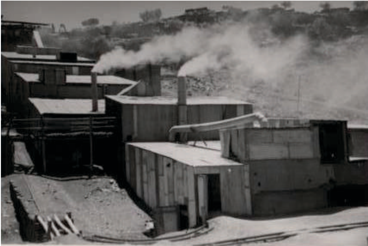
Typical discharge to atmosphere from an older plant. (‘Klipvlei’ written on the back of the photograph)
