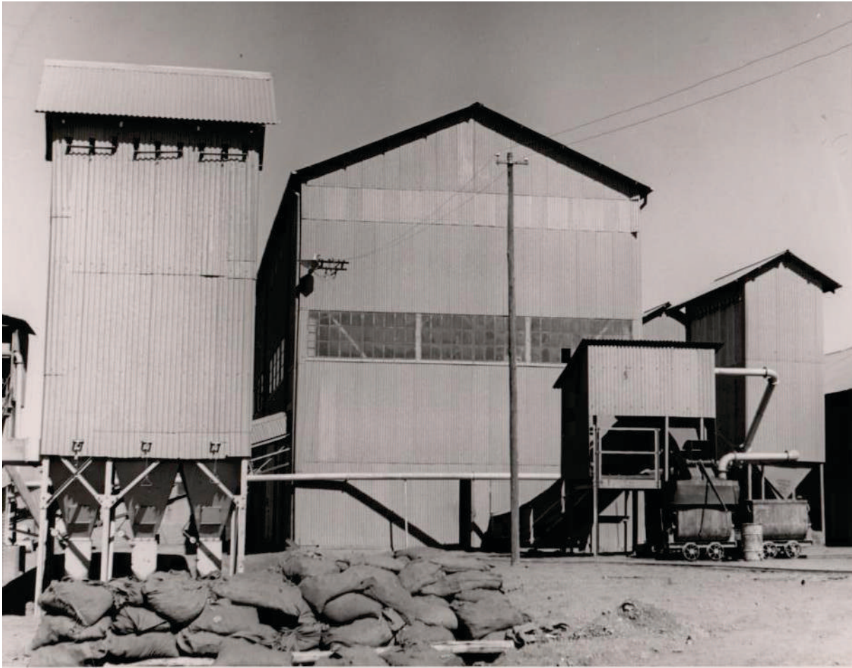
Prieska mill, or treatment plant
