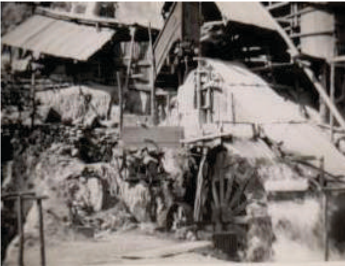
Waterwheel driving the first mill at Msauli
