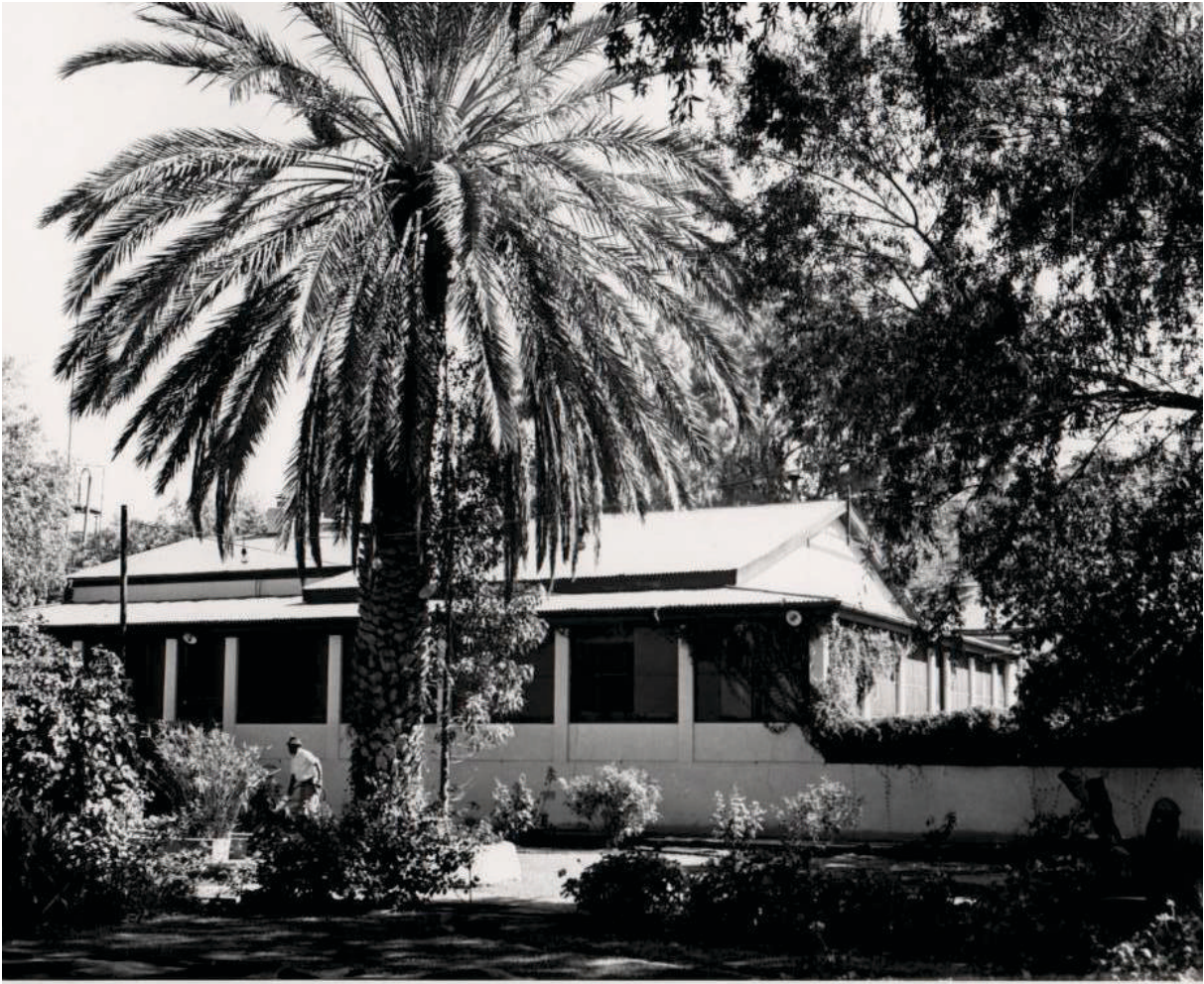
Mine Manager's residence, Koegas
