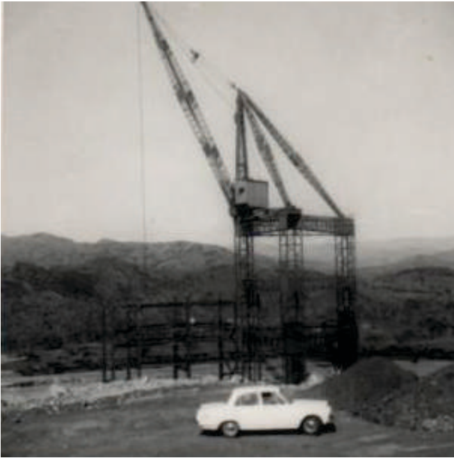
Crane to erect Msauli's new 11 storey mill building on site
